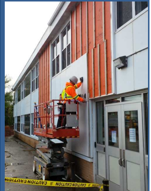
Renovations have begun!
